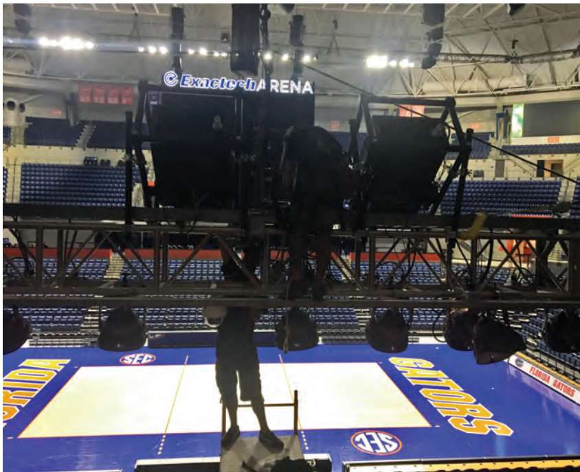
Quince installed Christie Boxer projectors in the center of the existing lighting truss on both left and right courts.
