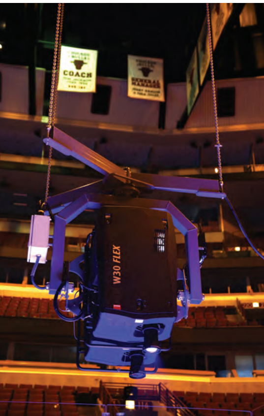
Rigging is a critical component to successful projection system installation. This Barco HDF w30 projector, installed at optimal trim height, ensures operational excellence and seamless in-game display.
